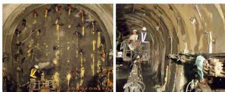
隧道開挖瓦斯洩漏封堵
